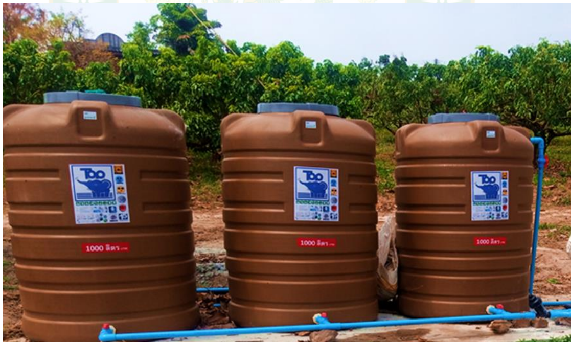
Figure 20 The tanks supplying water to the field.
