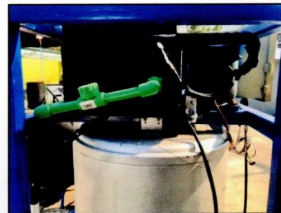
(b) The water box that installed at the evaporator section
